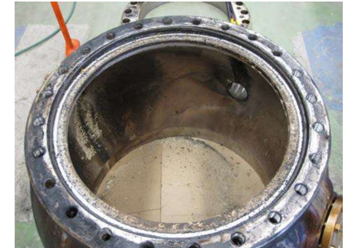
34. Carefully remove the seat ring. If stuck, please contact NAF for further instructions.
